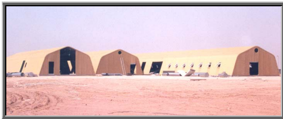
USAF Kitchen/Diner complex for 372 PSAB Saudi. Airfreighted in and erected by Military personnel
